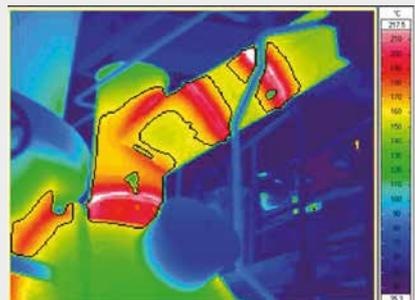
Left: Deficient insulation on a bypass line at a combined heat and power plant. Heat control faults are possible.
