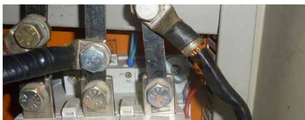
Fig. 1: Terminal of a power circuit breaker, inappropriate connection
