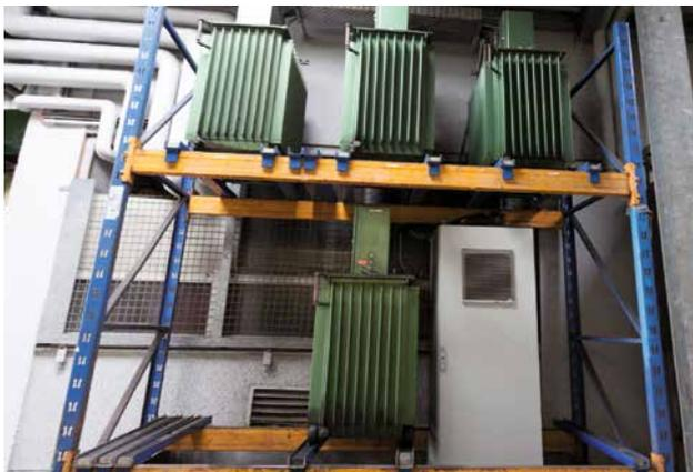
**Fig. 8:** Four rectifiers of 8 V 600 A each, with 215 kg oil for cooling. The missing separation of rectifiers with a fire rating creates the danger of fire spread into adjoining rooms. In addition, setting up and operating the rectifiers in shelves creates the danger of underfiring. For this reason, the rectifiers should be set up on level ground and at a minimum clearance of 2.50 m from one another as well as free of fire loads.
