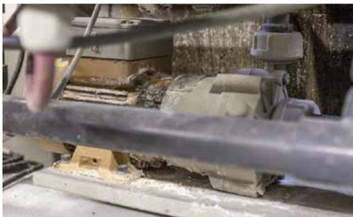
**Fig. 9:** Salt deposits on the metal housings of electric equipment result in both accelerated corrosion and overheating by restricted cooling.
