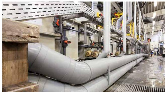
Fig. 6a and b: Fume extraction ducting as well as plastic equipment and supply units of electrolyte baths contribute to quick fire spread in the entire area of use in case of fire.
