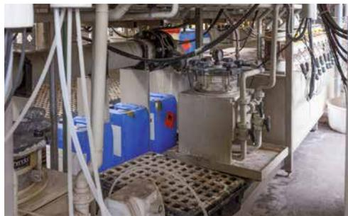
**Fig. 10a:** Open storage of flammable chemicals and solvents can also contribute to fire spread and should be avoided as a basic rule.
