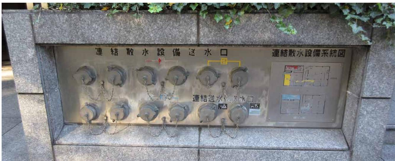
the fire department's initial response, it is recommended to provide a supply point within 80 to 150 meters of the property. For a quick response the firefighting water points should have a hose couplings, that can be used by the local fire department.
