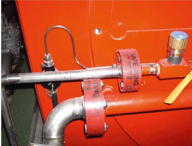
Fig. 2: Spray protection sleeves on oil flanges
