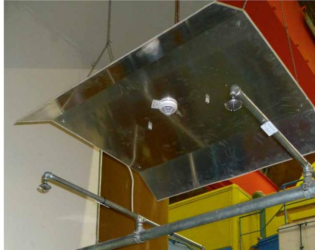
Fig. 7: Smoke detector with heat accumulation plate
